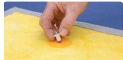
2 ▶ Insert marking plugs into the Snap-On Anchors*.
