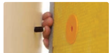
5 ▶ Firmly push panel onto ratchets to complete installation.
