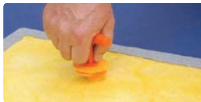
1 ▶ Screw Rototast Snap-On Anchors into the back of the panel using the rototast chiver tool.
